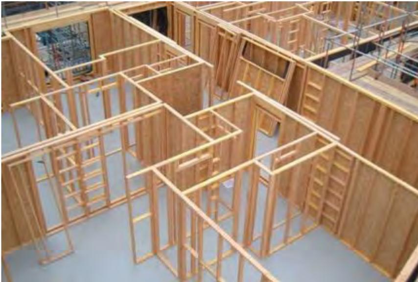
Figure 8 – Typical platform-framing (AFPA, 2001)
