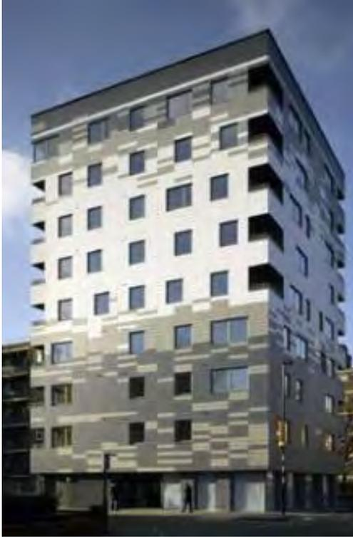
The prefabricated CLT panels allowed a team of four carpenters to construct the super-structure in less than four weeks (Waugh, Wells, & Lindegar, 2010).
