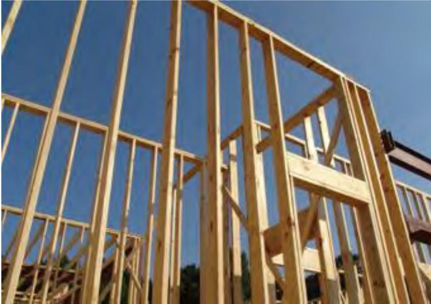
The light timber framing elements, also referred to as studs in walls assemblies and joists in floor assemblies, are used to form the internal and external partitions for the structure (AFPA, 2001). Timber studs are quickly assembled to frame the structure, with mechanical services and insulation located within the light timber frame assembly.
