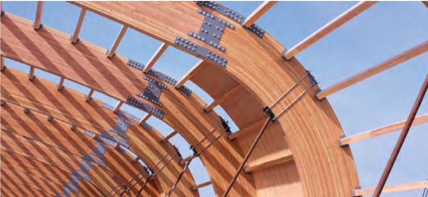
Figure 30 – Glulam beams (WoodSolutions, Glulam, 2013)
