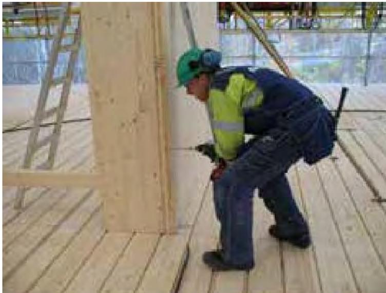
Panels and boards are attached to timber elements using nails and screws. The following images show examples of gypsum board framing to timber elements.
