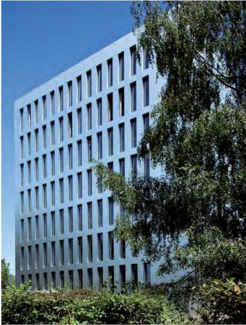
The Life Cycle Tower structural design is based on post and beam construction with large internal and perimeter glulam columns. These are combined with a concrete core for stability and hybrid timber-concrete floor slabs for fire separation and acoustic performance (Wurm, Gockel, & Unger, 2012).
