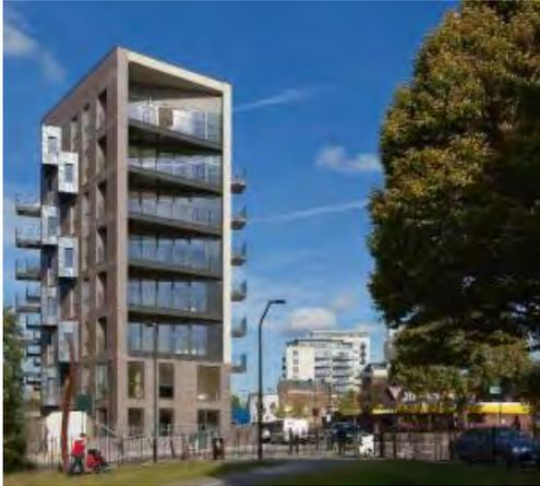
CLT construction was chosen over steel and concrete due to weight concerns as a storm relief sewer is located under the site. The use of CLT allowed the building to be lightweight, and prefabricated panelized construction resulted in a construction time of 10 weeks, less than half the estimated time for a concrete structure (Birch, 2011).
