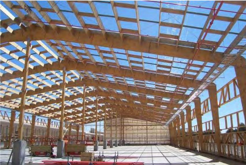
Figure 32 – Post and beam construction (Lignum, 2010)
