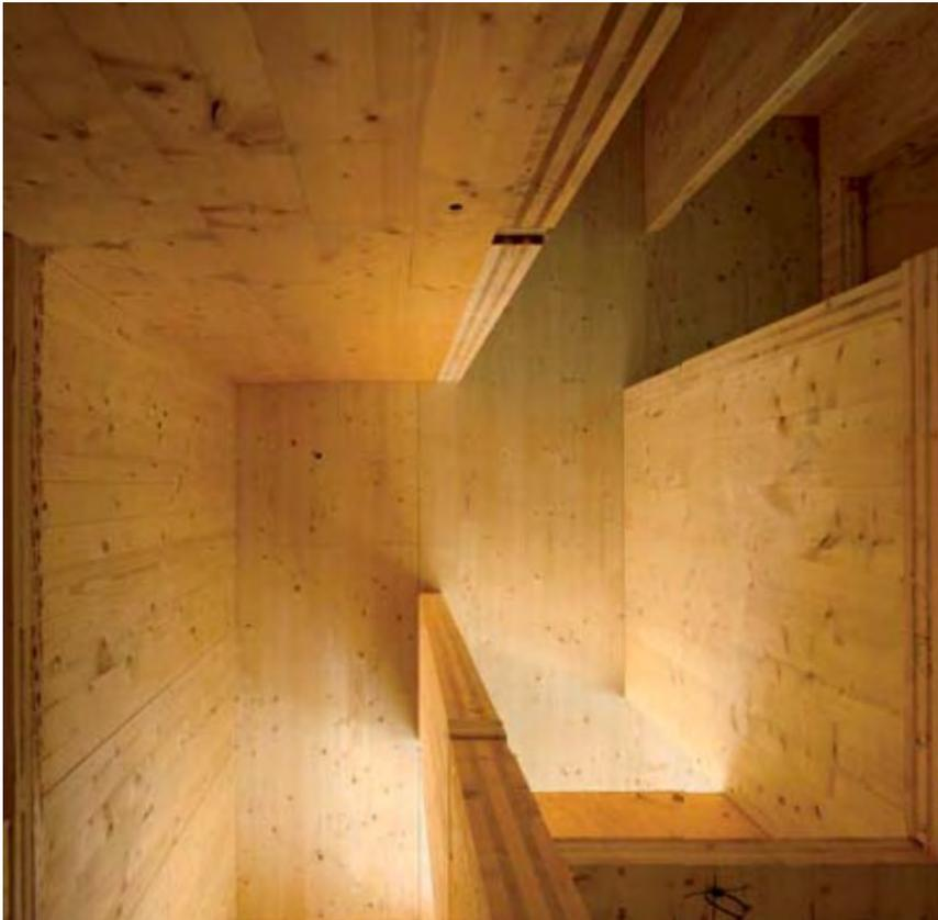
Figure 38 – Exposed CLT wall in Forté Building (FPInnovations, Cross Laminated Timber (CLT), 2013)
